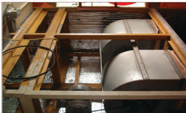
Innvendig Astro-Foil i aggregatet
